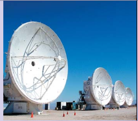
12-meter antennas of ALMA-Japan constructed at the ALMA Operations Support Facility in Chile
